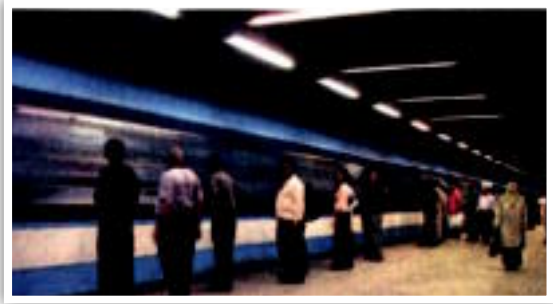
Fig (2-6): The fluorescent lamp are used to light the underground metro.
