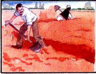
a) preparing the ground
