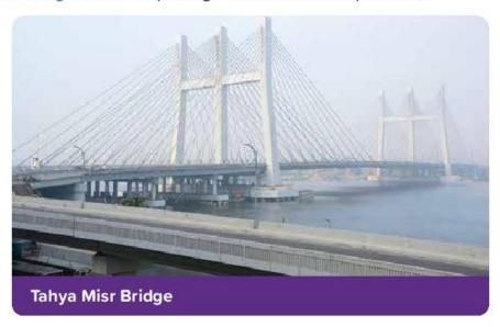
The Tahya Misr Bridge was built in 2016 in Cairo. It serves as a connector across the Nile from northern and eastern Cairo to western Cairo. The bridge is 540 meters long and 67.3 meters wide. It holds the world record for the widest cable-stayed bridge in the world.
