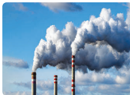
Figure (16) Pollution caused by combustion in industry
