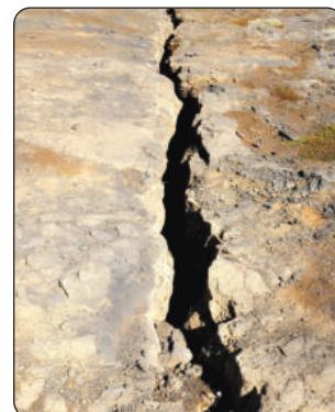
Figure (10) Earth crack
