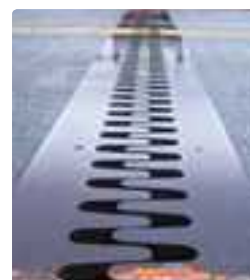
Expansion Joint on Bridge
