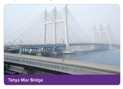
The Tahya Misr Bridge was built in 2016 in Cairo. It serves as a connector across the Nile from northern and eastern Cairo to western Cairo. The bridge is 540 meters long and 67.3 meters wide. It holds the world record for the widest cable-stayed bridge in the world.
