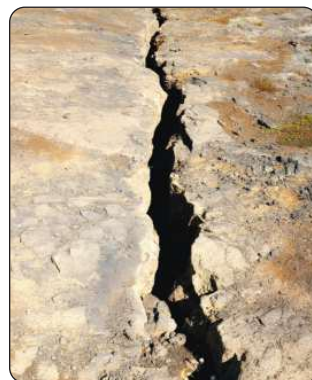
Figure (10) Earth crack
